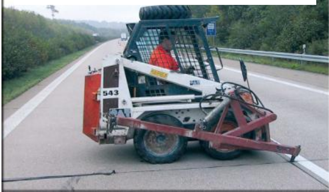
Removing old Joint Sealant
