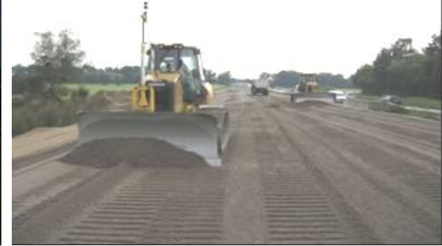
Placement with Finisher or Grader
