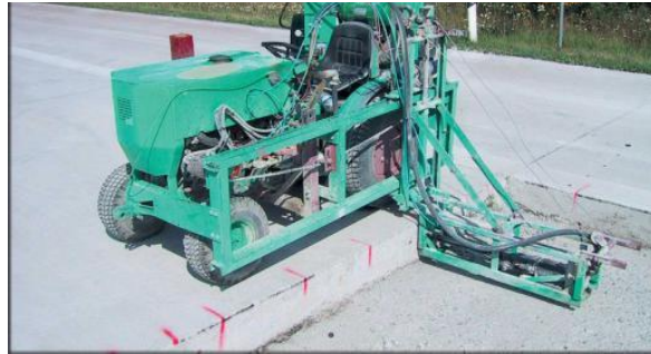
Drilling machine for installation of tie-bars and dowels
