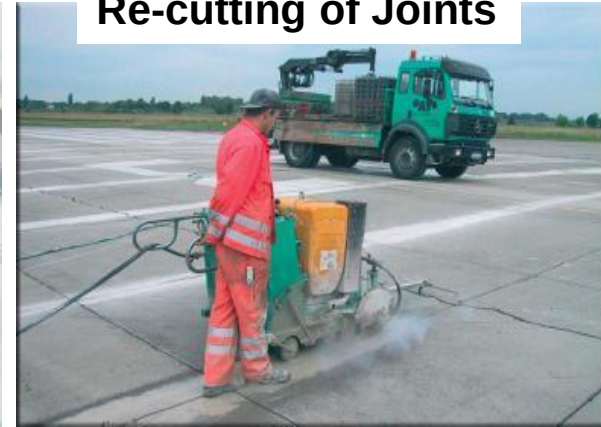
Re-Sealing of Joints
