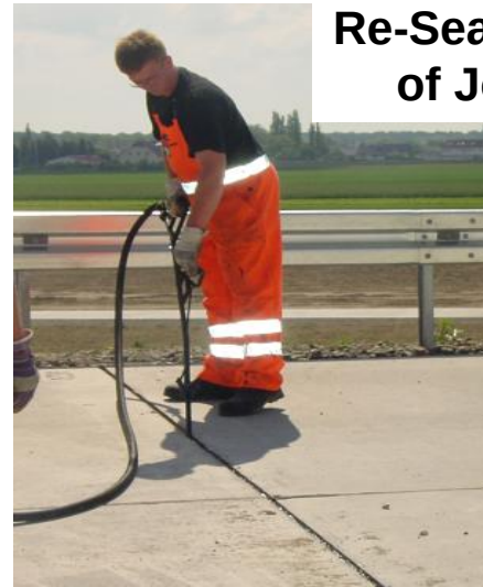
Installation of backer rod
