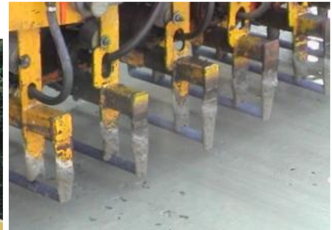
Placement of Dowel Bars
