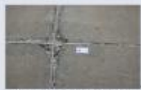
Figure 1: Concrete sealant in a joint.
